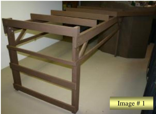
Basic wood benchwork with 1" x 4" "L" girders, joists and supports. Legs are 2" x 4"s bolted to the floor with metal "L" brackets. Carriage bolts hold the legs to girders.
